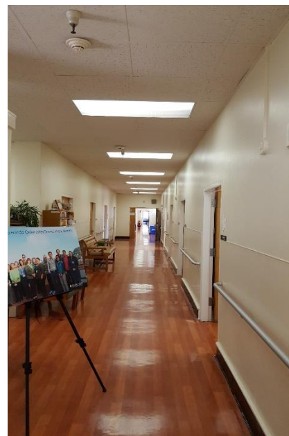
C-5 – Space Renovated for Medical Social Services
