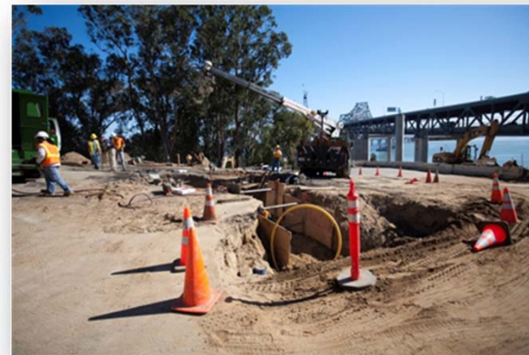
Treasure Island Pipe Relocation
