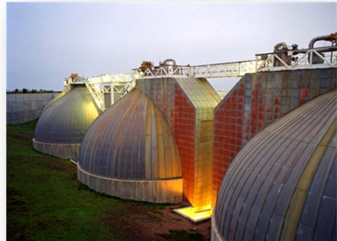
Oceanside Treatment Plant
