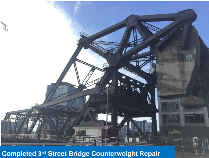
Repairing the 3 rd Street Bridge Counterweight
