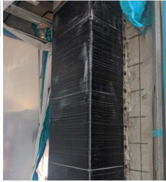
Seismic Upgrade – column strengthening w/ fiberwrap
