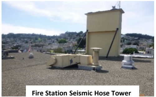
Fire Station Seismic Hose Tower
