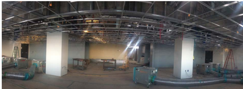
6H Surge (Ward 6H) – above ceiling utilities
