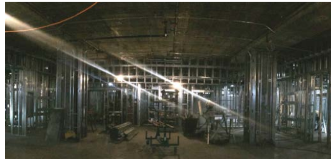
Rehab Dept Relocation (Ward 3G) – wall framing
