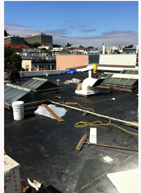
Roof replacement in progress at Fire Station 6
