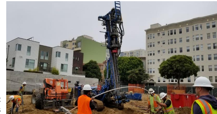
FS 5 Drilling and Placement of Soil Micropiles
