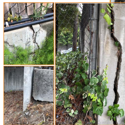
Cooling Tower foundation (above) structurally unstable.
