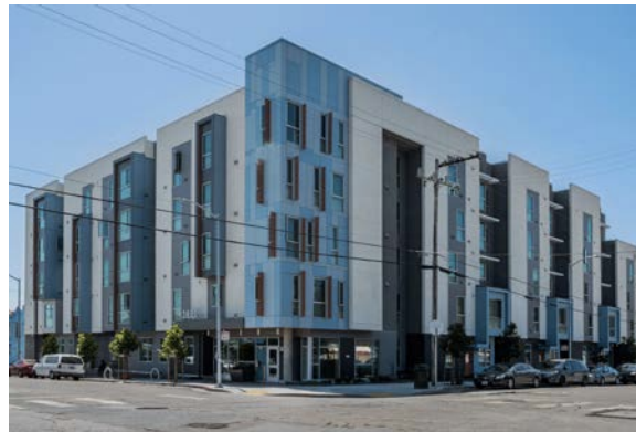
Completion of 700+ units through HOPE SF, including Sunnydale Parcel Q (District 10)
