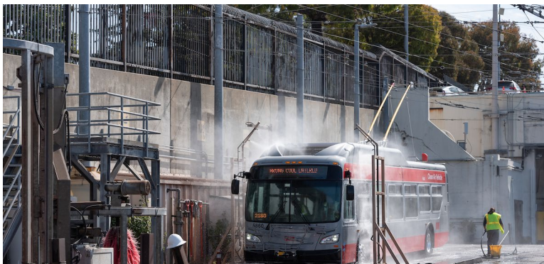
Bus Washers & Maintenance Bay Replacement
