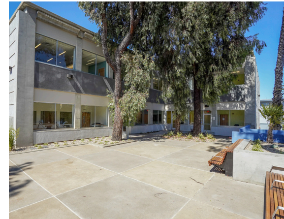
Castro Mission Seismic Retrofit
