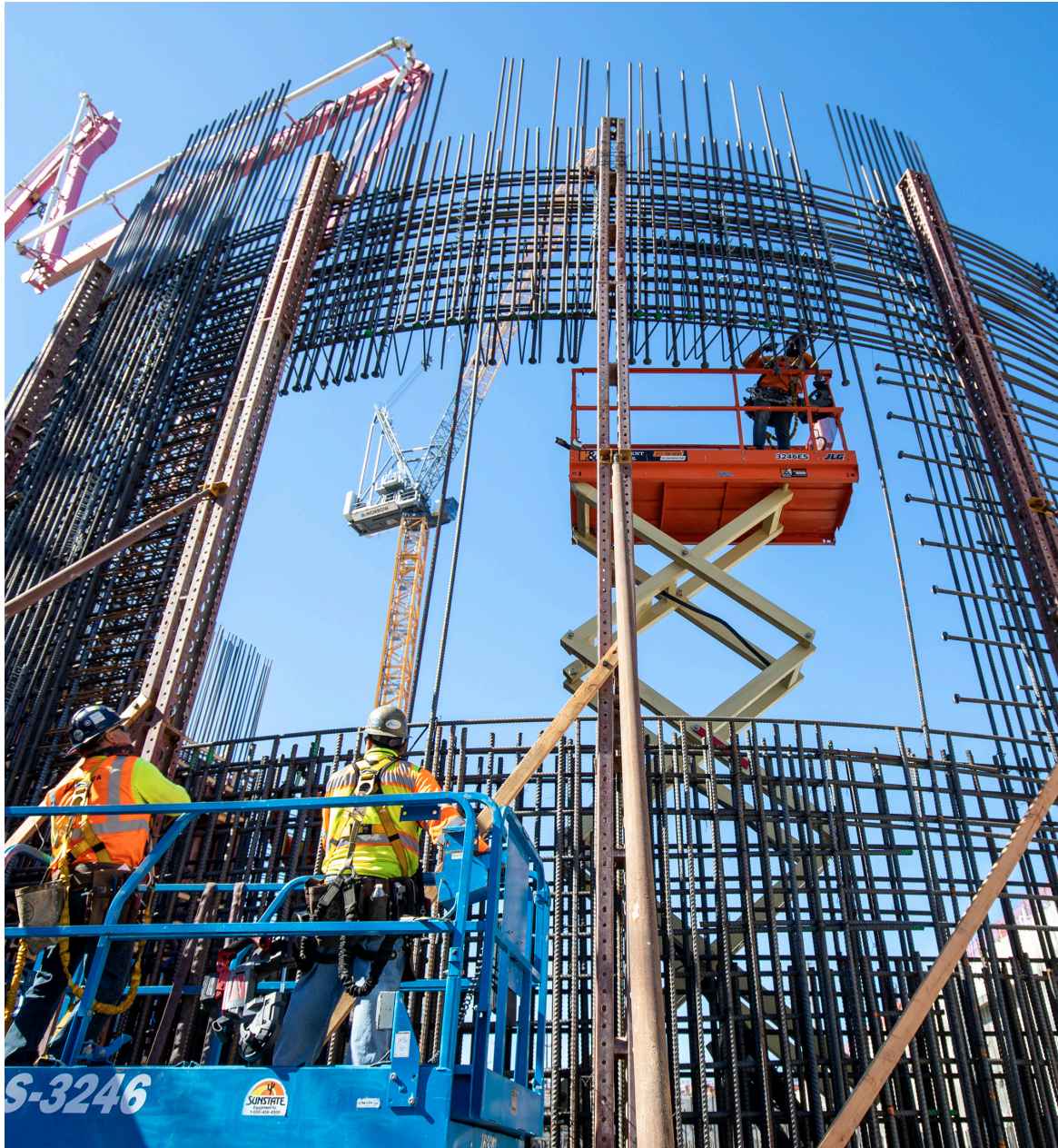
Biosolids Facility Construction
