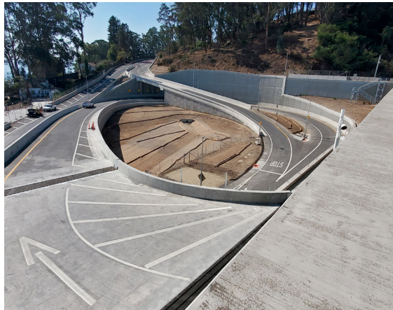
Treasure Island Southgate Road Realignment
