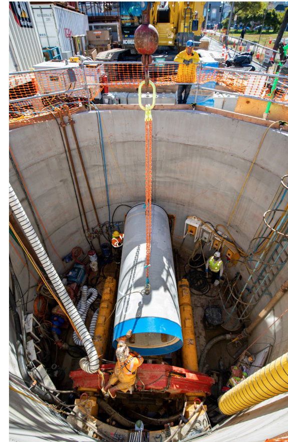
Construction at Wawona Vincente
