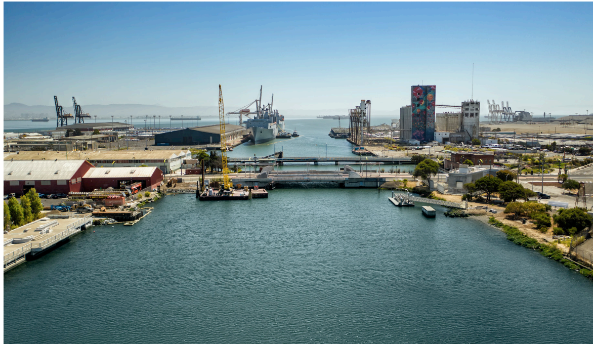
Islais Creek Bridge
