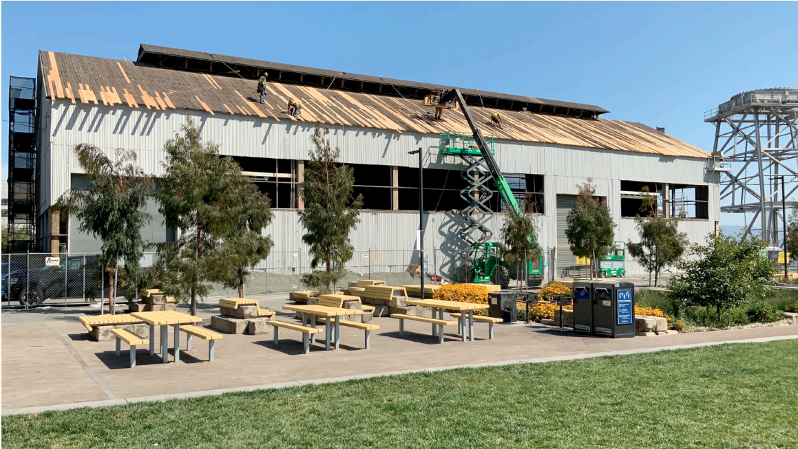
Roof Replacement at the Port
