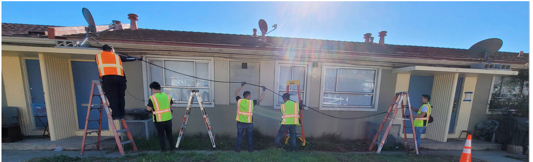
Fiber Broadband Installation
