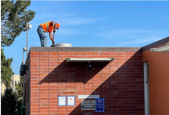
Marina Branch Library Waterproofing
