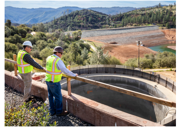
Mountain Tunnel at Hetch Hetchy
