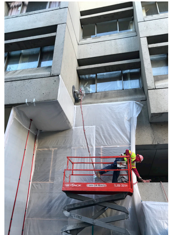
Building 5 Seismic Upgrade
