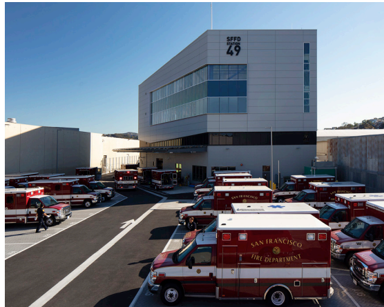
Fire Station 49 and Ambulance Yard
