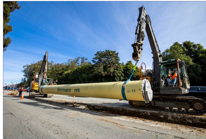
36-inch PEWFS Pipeline at 19th Ave and Sloat Blvd
