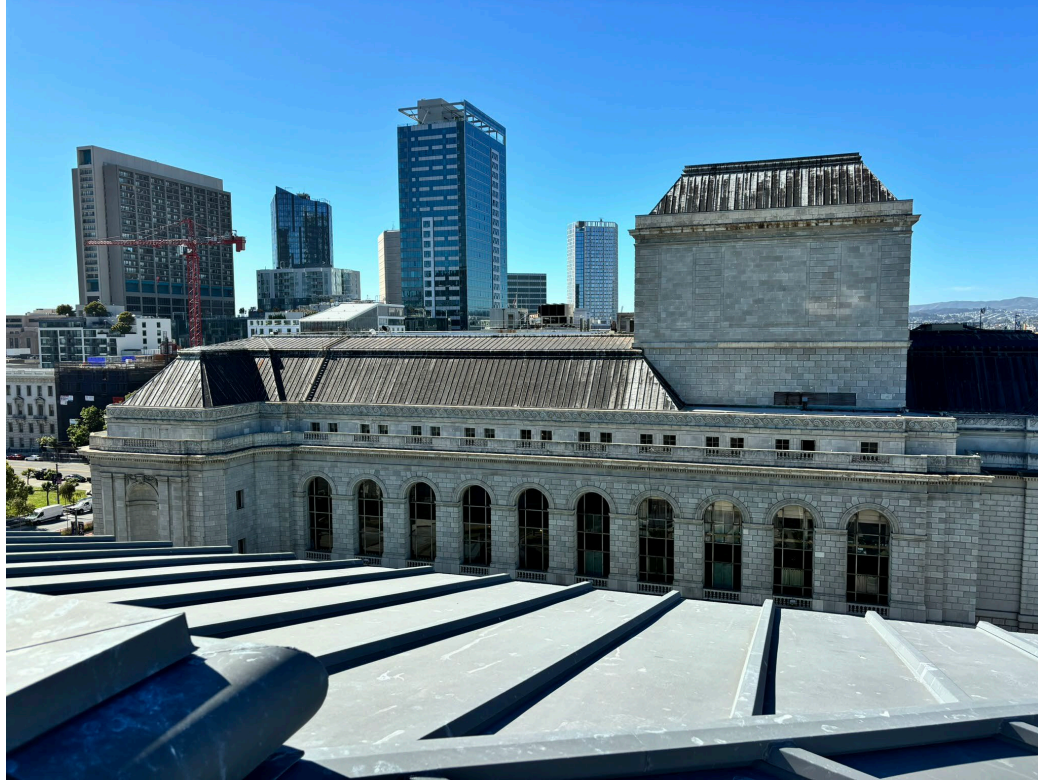
Opera House Roof Replacement
