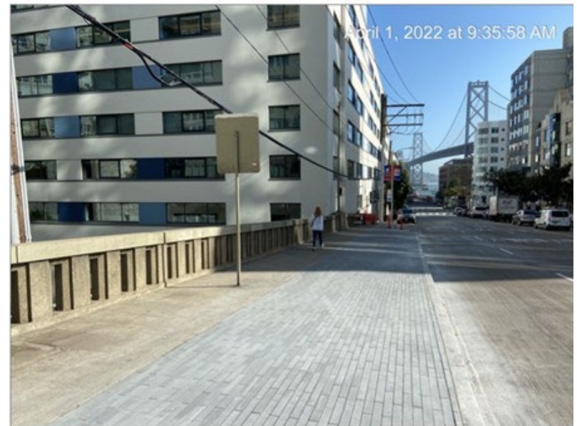
Harrison Streetscape – Beale Street Bridge
