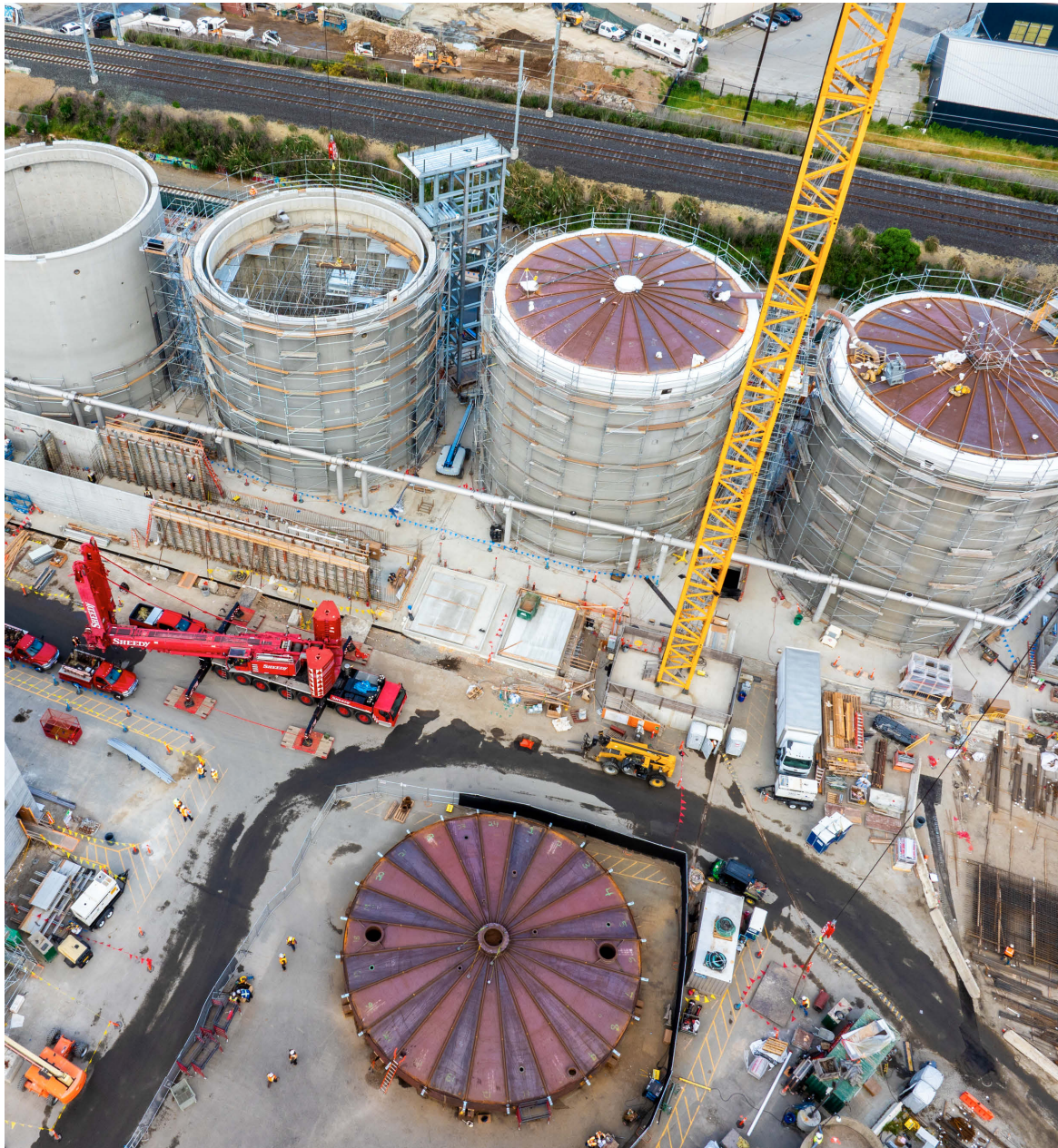
Biosolids Digester Project
