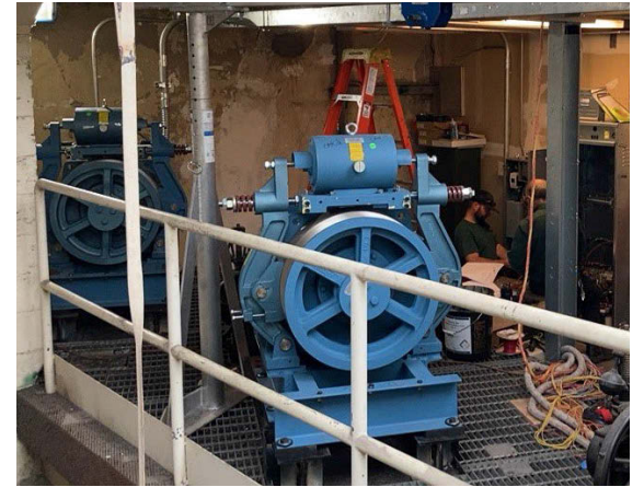
City Hall Elevator Modernization
