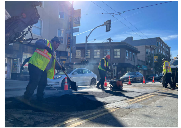
Pothole Repair
