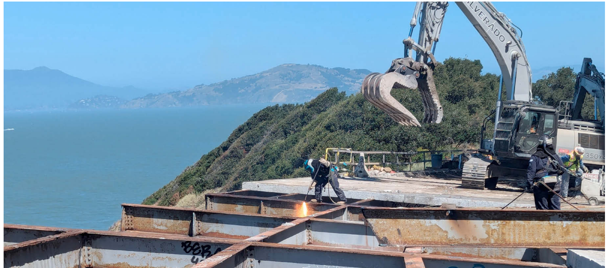
Yerba Buena Bridge Construction
