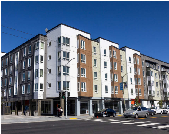
4840 Mission Street Bridge Housing
