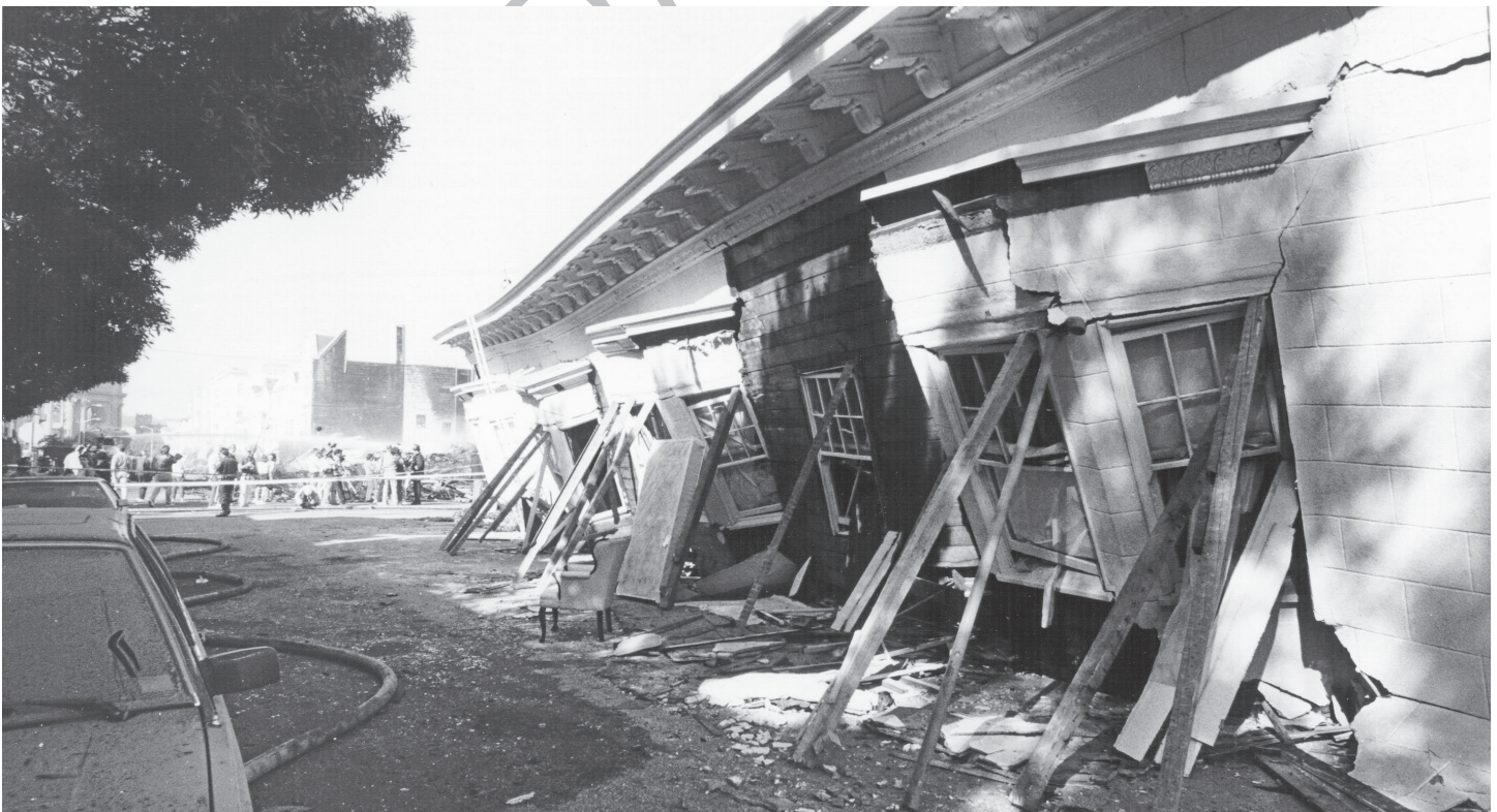
Aftermath of the 1989 Loma Prieta Earthquake
