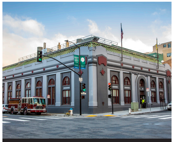
Emergency Firefighting Water System: Pump Station No. 1
