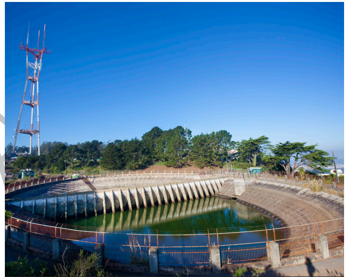
Emergency Firefighting Water System: Twin Peaks Reservoir
