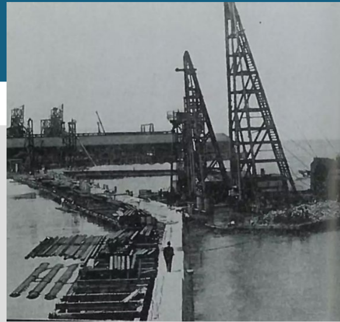
Embarcadero under construction
