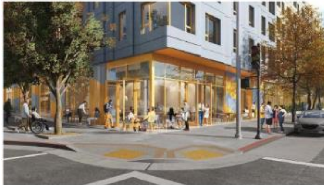
730 Stanyan Completed in 2025
