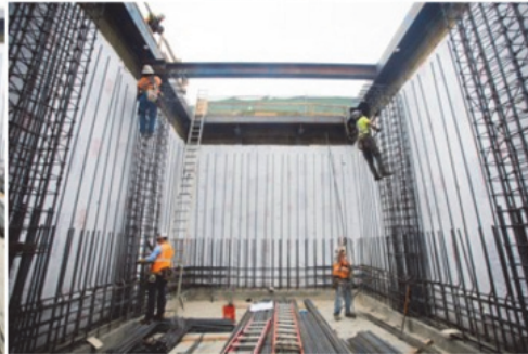
Figure 2-22 New cisterns under construction (image from http://slideplayer.com/slide/10267606/ )
