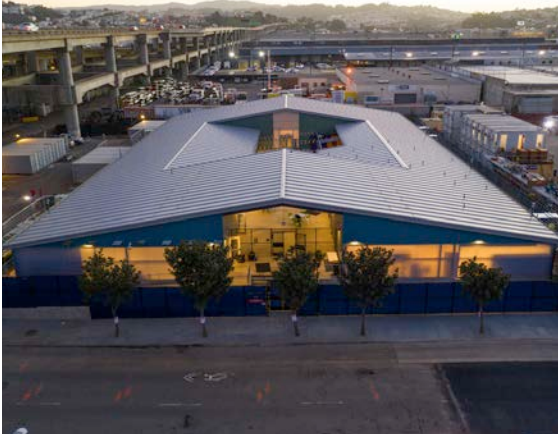
Bayview SAFE Navigation Center
