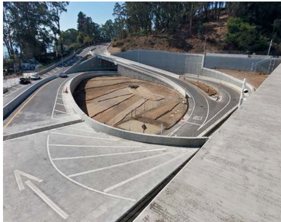
Treasure Island Southgate Road Realignment
