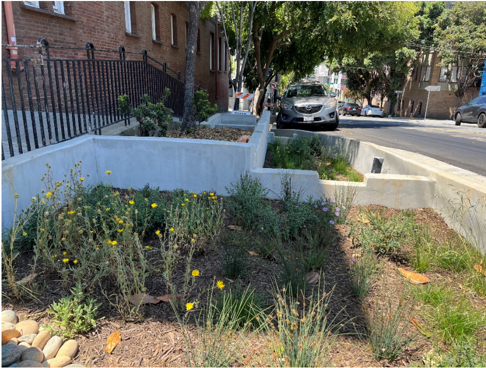
Green Stormwater Infrastructure on Page Street
