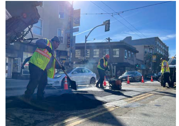
Pothole Repair
