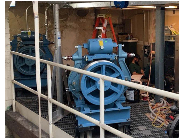
City Hall Elevator Modernization
