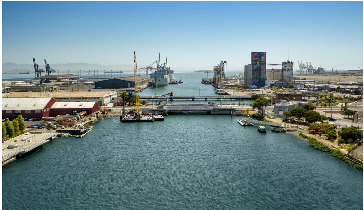
Islais Creek Bridge
