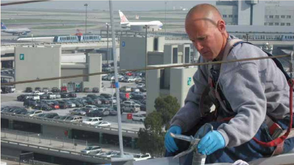
Roof Repair at SFO
