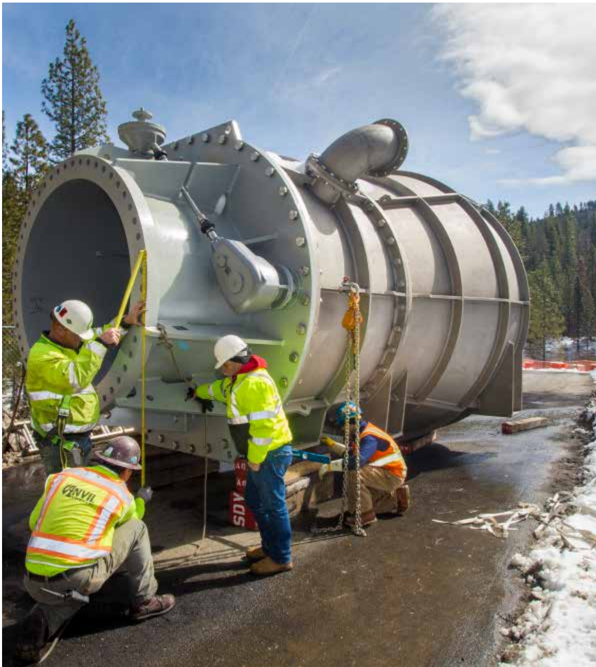
Cherry Dam Outlet Works Rehabilitation
