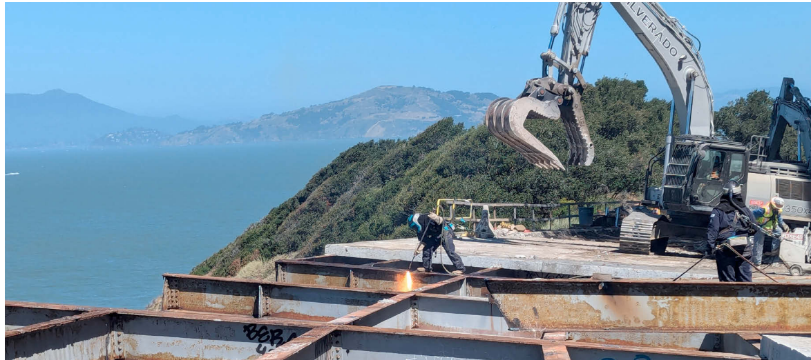
Yerba Buena Bridge Construction
