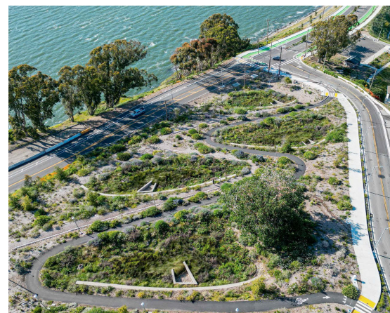
Treasure Island Infrastructure
