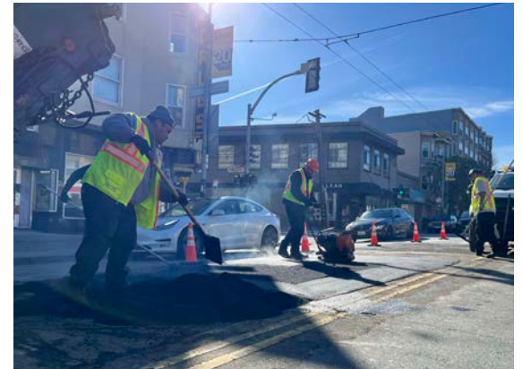
Pothole Repair
