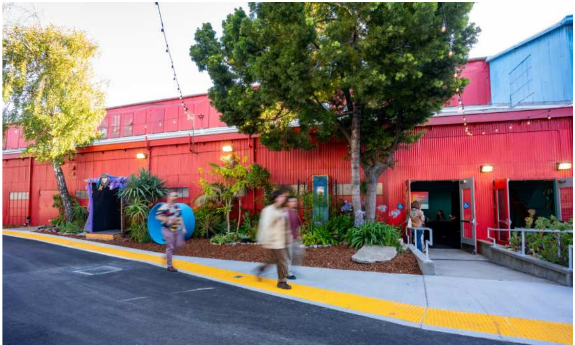
SOMArts Exterior ADA Barrier Removal and Retaining Wall
