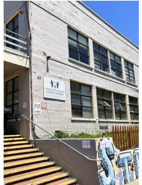
50 Raymond Street Siding Repairs
