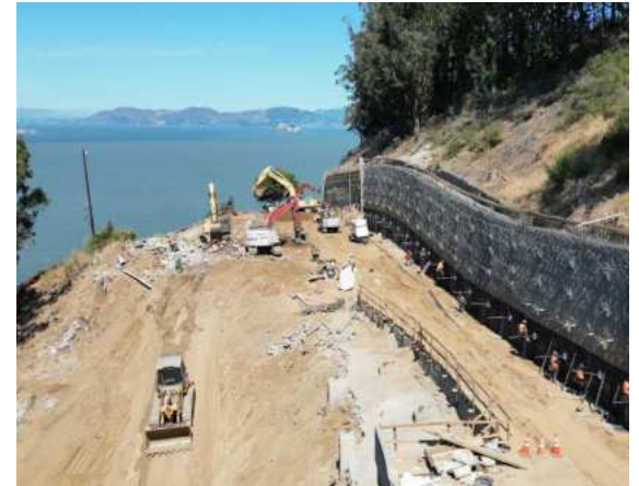
Yerba Buena Island Bridge Construction
