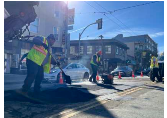
Pothole Repair
