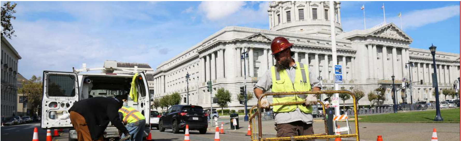
Civic Center Steam Loop Repair
