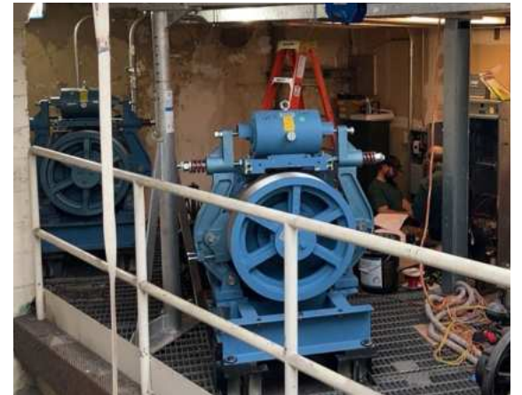
City Hall Elevator Modernization
