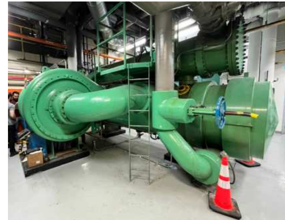
HOJ Chiller Replacement
