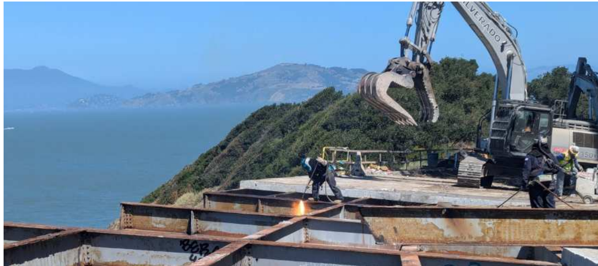
Yerba Buena Bridge Construction
