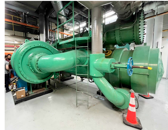
HOJ Chiller Replacement
